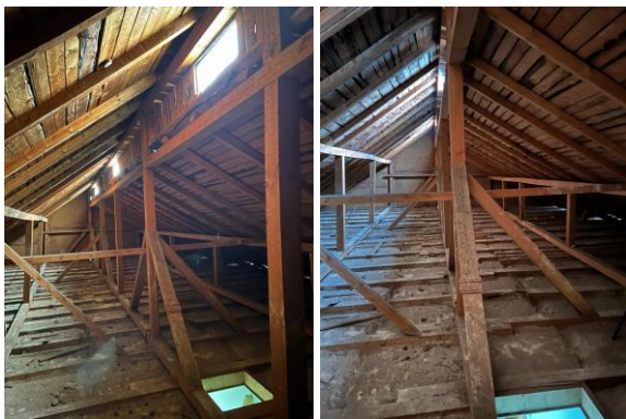
Figure 2 Details of the trestle frame roof studied.
