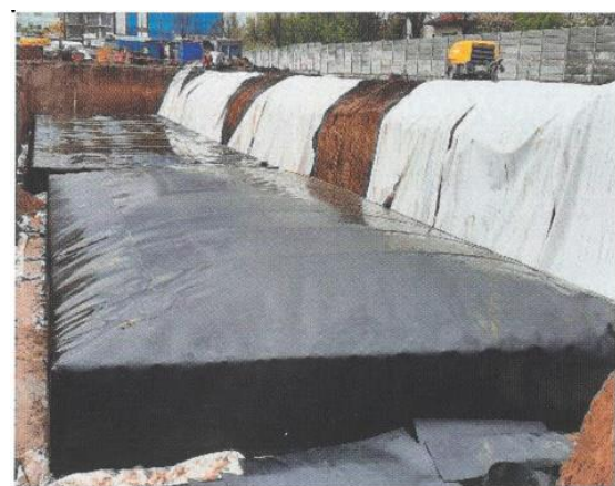
Figure 6 Carrying out the tightness test with compressed air [12]
