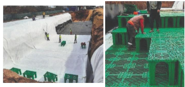
Figure 4 Stages in the realization of modular tanks [12]
